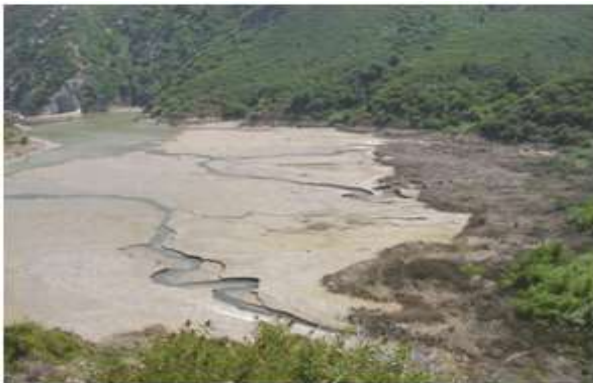
Fig. Matilija Dam on the Ventura River (USA), height 65 m, reservoir capacity 8.6 million m 3 (over 65 years, 95% of the volume has been filled with sediments)
