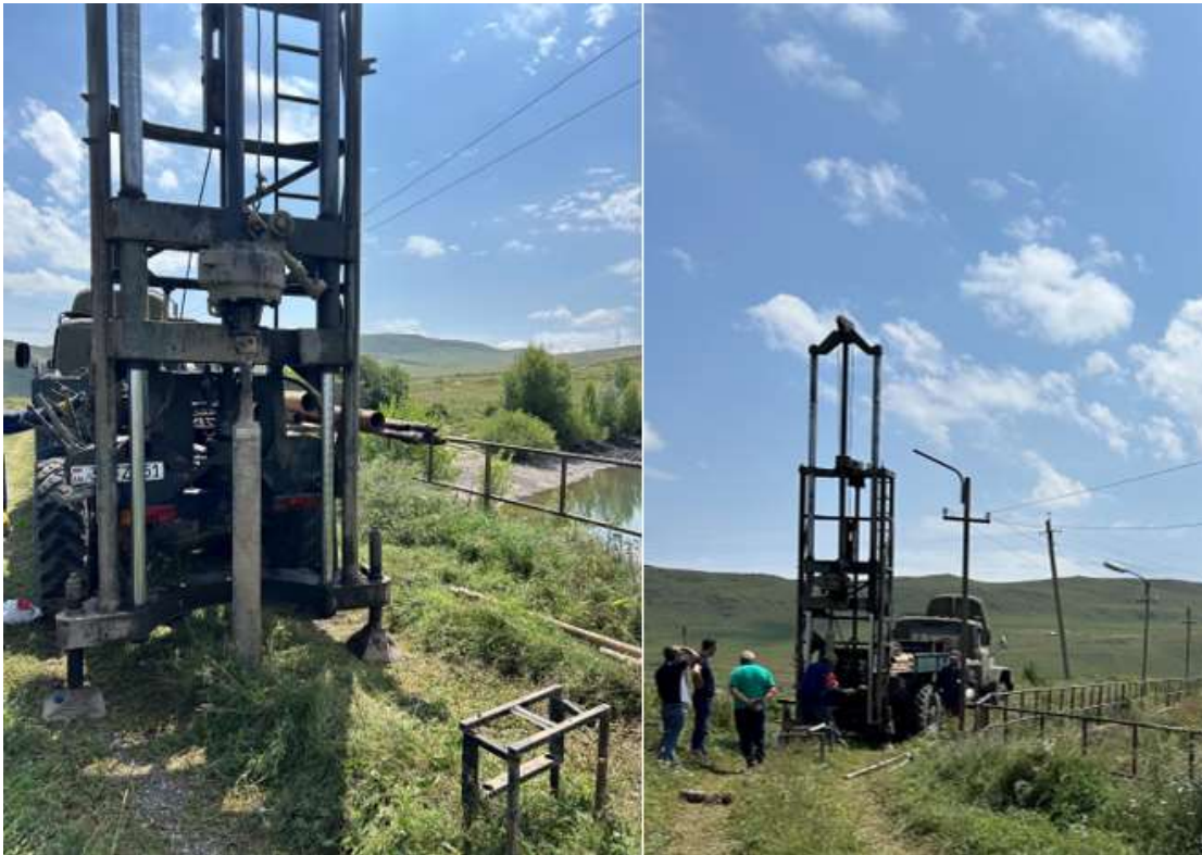
Fig. 1 Drilling of two wells in the body of the dam «Gegharkunik 2»
