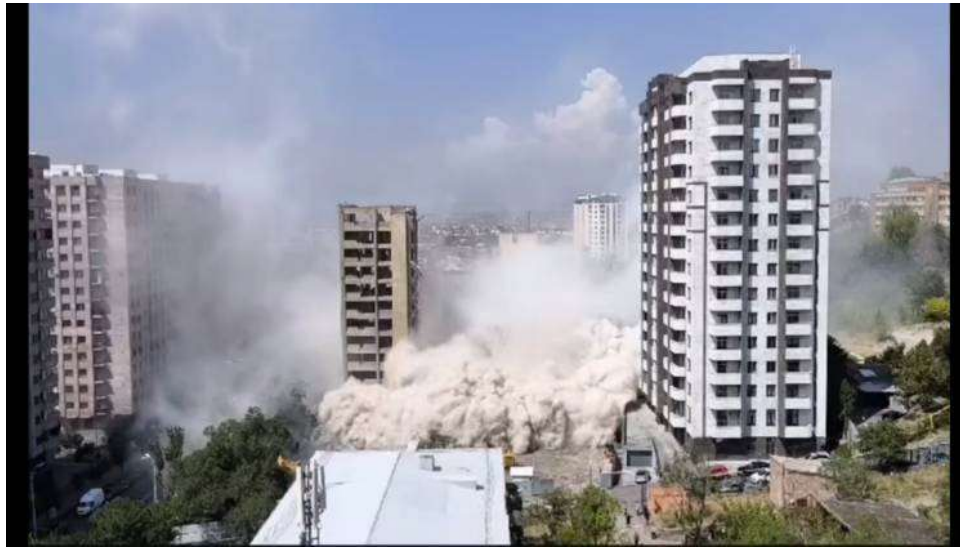
Fig. 4 The process of dismantling the building in Yerevan, 2024.
