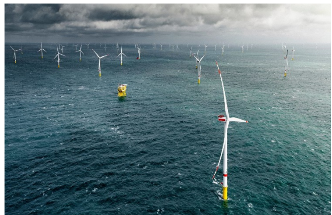
Pic. 3 Hornesa offshore power plant in England
