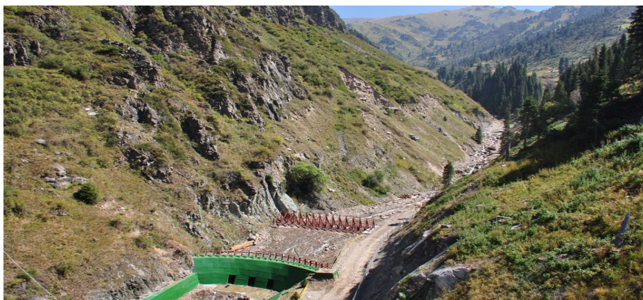
Fig. 1 Cascade of mudflow protection facilities: downside monolithic – made of reinforced concrete, upside– made of collected metal constructions.
