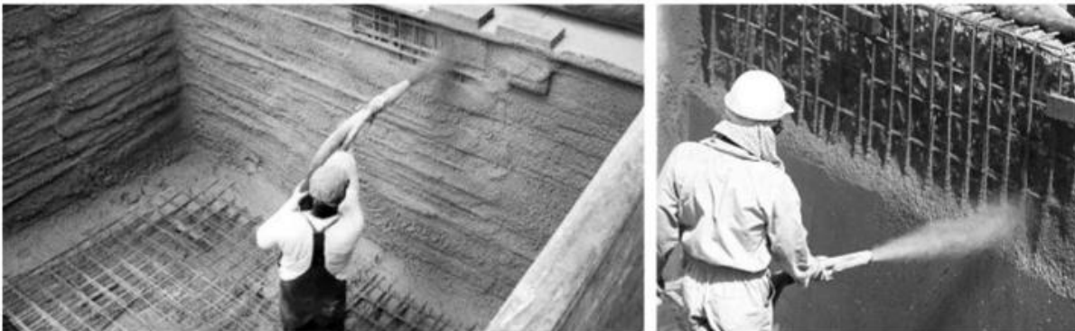
Fig. 3 Shotcreting process
