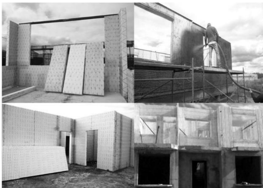
Fig. 4 Window and door parts installation
