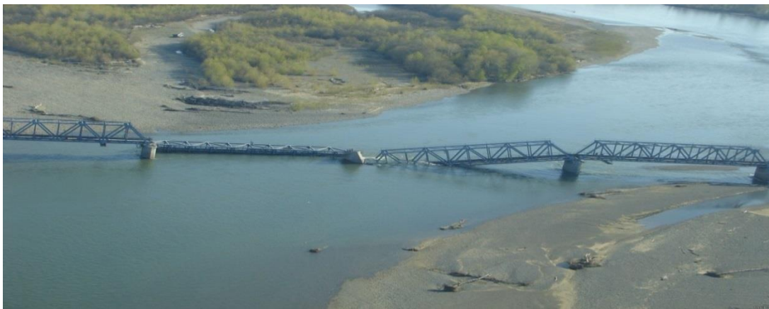
Figure 3. Failure of bridge supports caused by flood
